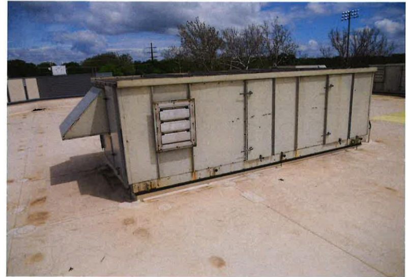
1983 Maintenance Bay Ventilation Equipment (HRU-1) (Installed in 1983; currently 37 years old)
